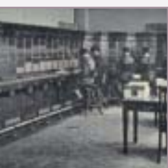
Original telephone exchange, Imperial Chemical House, 9 Millbank, London SW1
