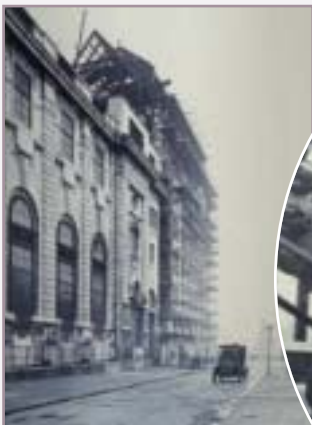
Construction of Imperial Chemical House, 29 January 1928
